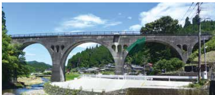
6 (廢)幸野川橋梁
